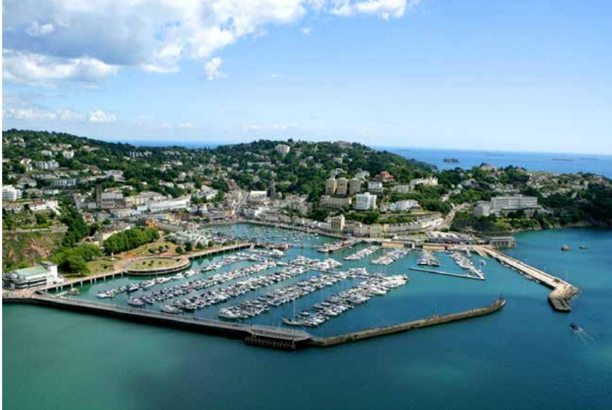
of its seaward face as well as raising the breakwater's height by 50cm is expected to substantially improve its utility as a breakwater and future-proof it against rises in sea level due to climate change for up to 50 years.
